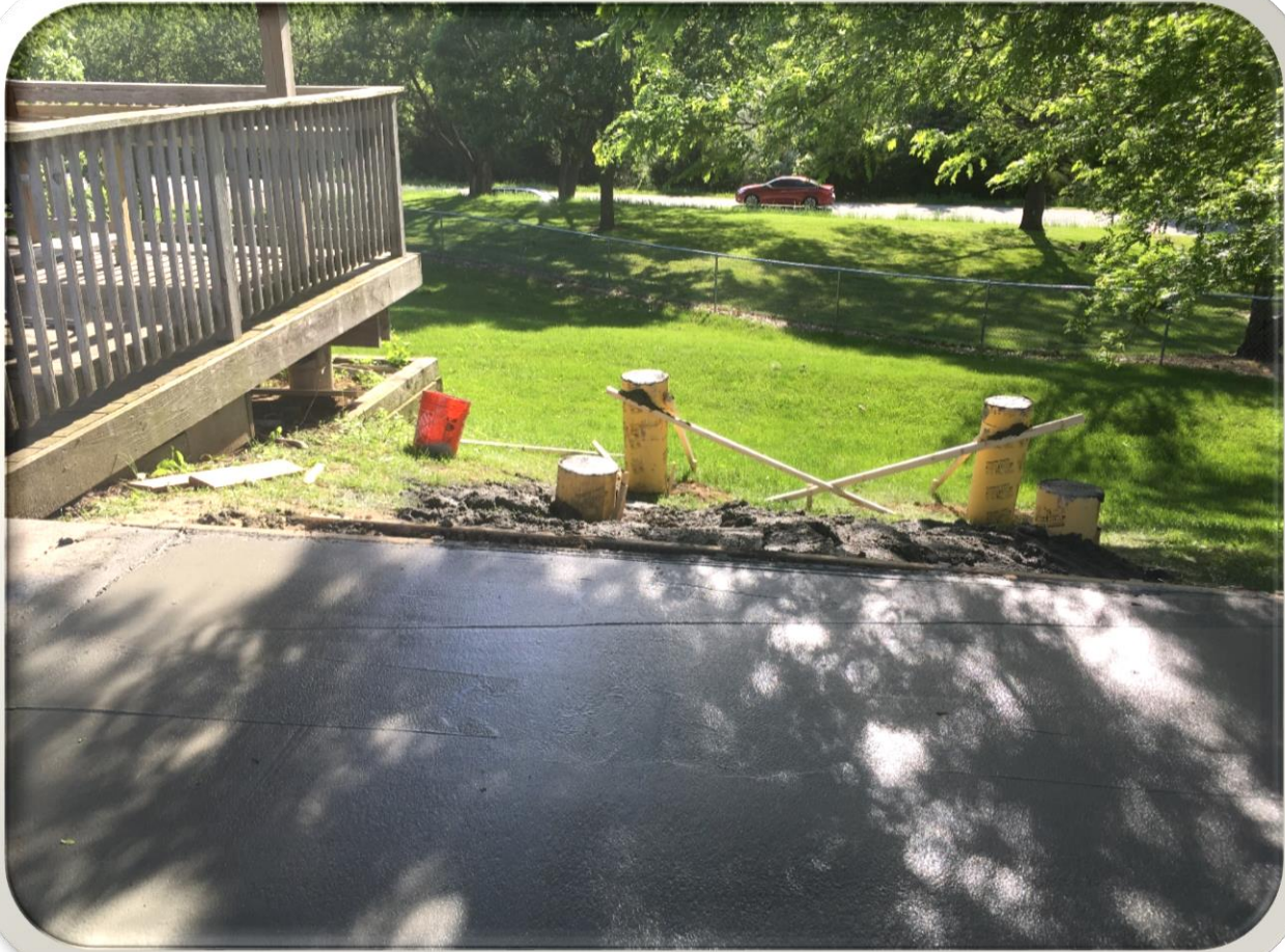
New Pad being poured adjacent to existing structure
