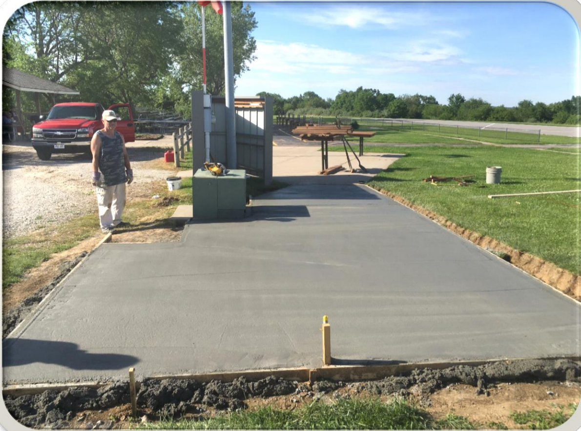
Ron B, inspecting the New Restroom / Maintenance Pad
