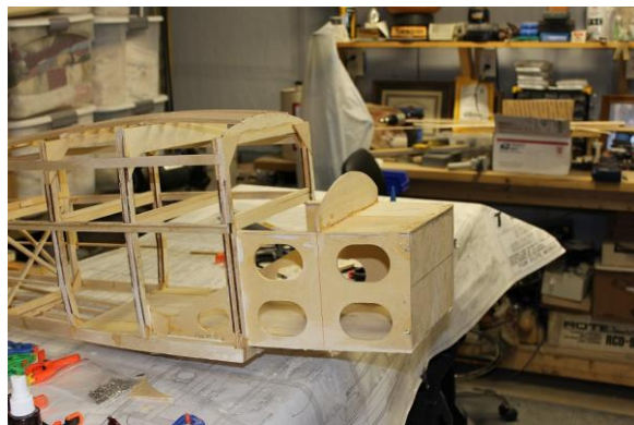
Former F-2 added to nose structure
