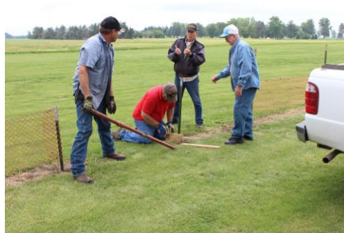
Removing post to enlarge gate to runway
