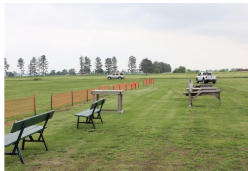
New section of safety fence complete
