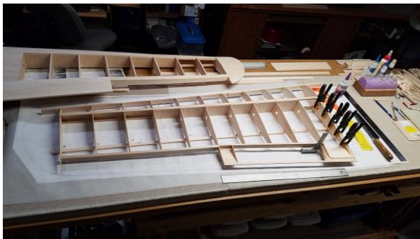
Top view of wing before sheeting. Shows the exposed cavity that will hold the left wing flap.
