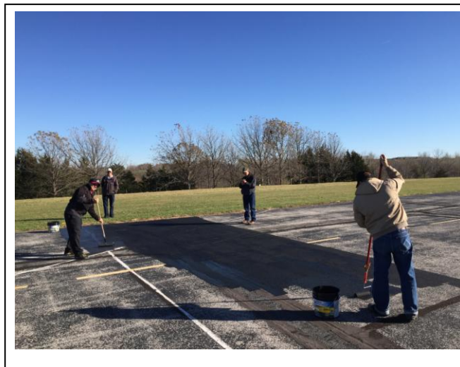
Gary Vohnout, Larry Inness, John Thompson, and David Haney putting down a test strip of asphalt sealer this past week.
