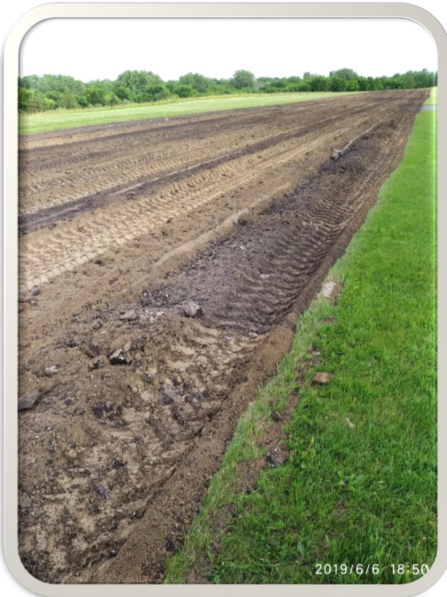
Old runway surface is removed down to earth!
