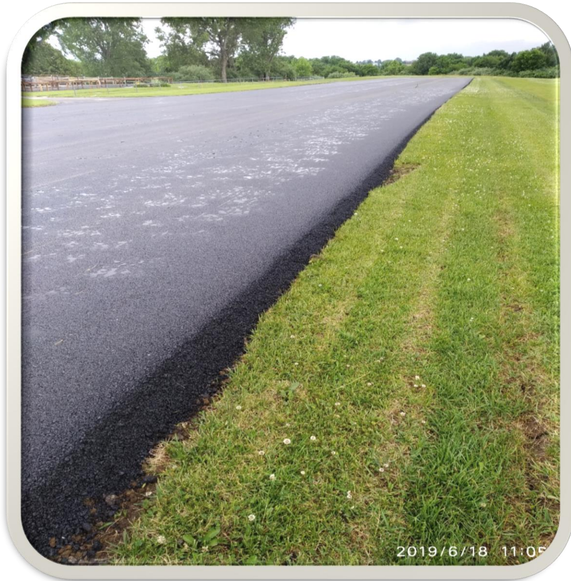
The finished product, awaiting final painting
