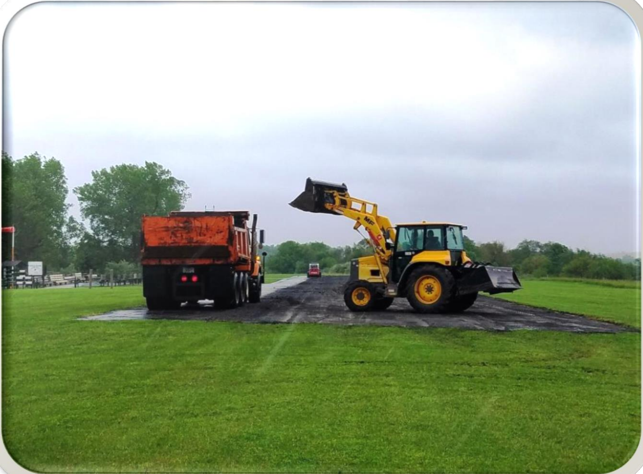
Removal of the top surface of Runway in progress
