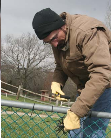
Erik patches the safety fence
